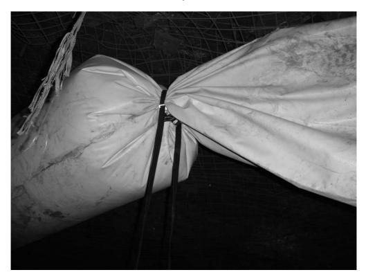
Picture 10. An example of closed air tube
